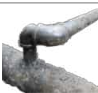
2. Street Elbow on a TOE Nipple
