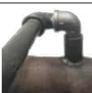
3. Street Elbow on a Coupling
